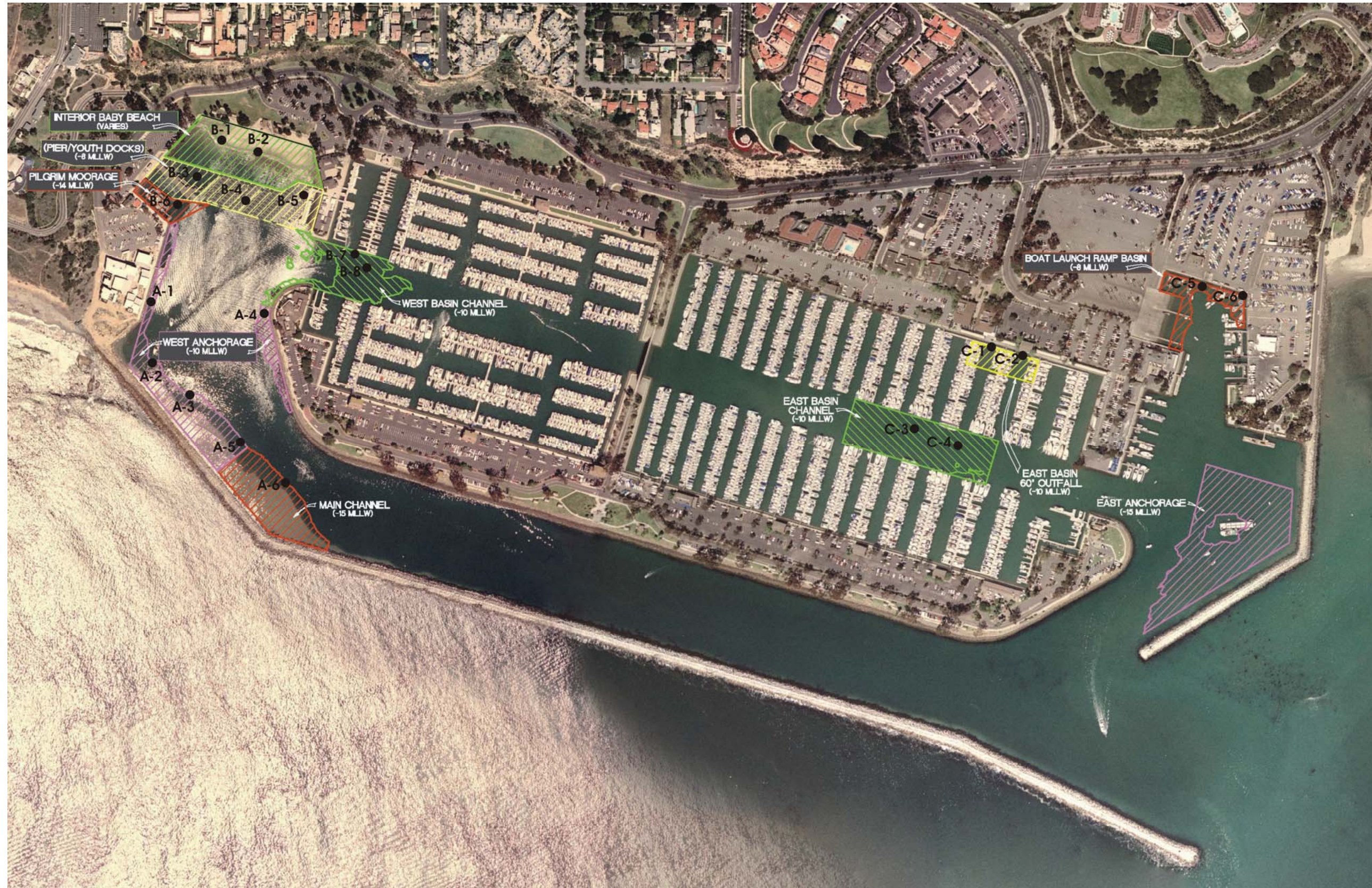
Figure 2. Dana Point Harbor Limits of Dredging and Final Sampling Locations
